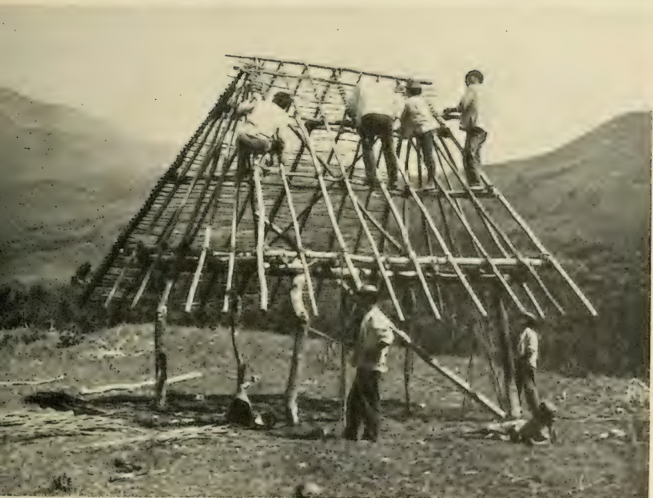
PLATE 39.—Hip-roofed house of the Guaymí. Top: Completed. Bottom: Framework. (Courtesy Frederick Johnson.)
